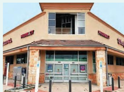
This Walgreens store in Texas was damaged in Hurricane Harvey.
