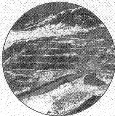
Andina Expansion Project, Chile Environmental impact statement to expand copper production in the Valparaiso and Santiago Metropolitan Regions.
