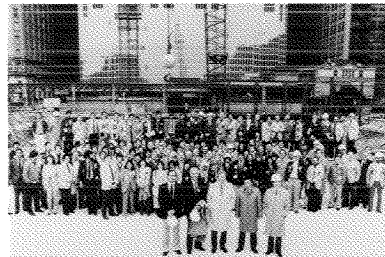
1981 CBOE breaks ground on a 350,000-square-foot building across the street from the Chicago Board of Trade.
