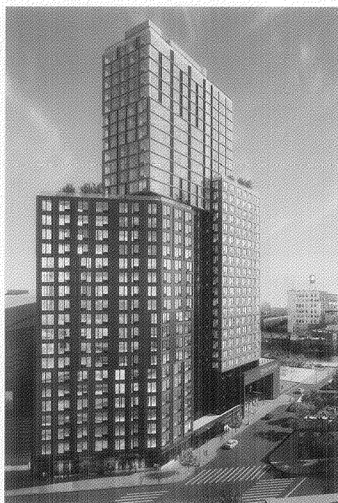
Adjacent to Barclays Center, B2 BKLYN is currently under construction and will be the first residential tower at Atlantic Yards. Using a modular construction process, the 32-story tower will feature 363 units, half of which will be reserved for low-, moderate- and middle-income households. B2 BKLYN is expected to be the first project to be part of our strategic capital partnership with the Arizona State Retirement System.
