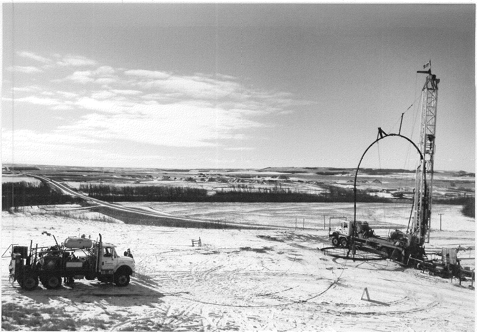
Weatherford COROD® continuous rod deployment in a heavy oil well, Northeastern Alberta.
