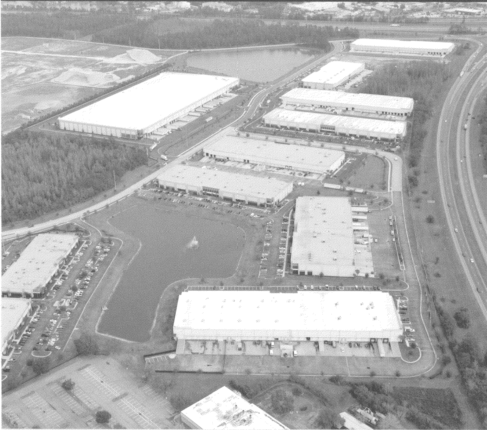
Southridge Commerce Park, Orlando, Florida
