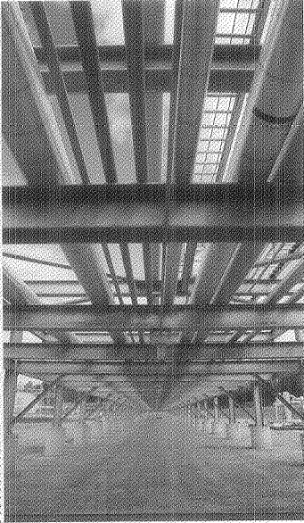
Tinsley EOR facility
