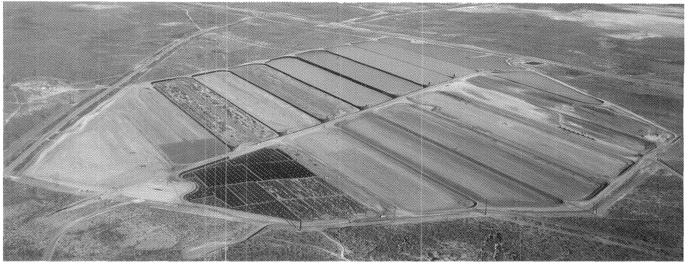
Aerial view of HB solar evaporation ponds.
