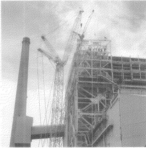
Construction of an emission control project at the Edgewater Generating Station Unit 5 in Sheboygan, Wis. was completed during 2012. When combined with an earlier project, we have reduced nitrogen oxide emissions by approximately 65%.
