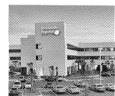
Brooksville Regional Hospital Brooksville, FL
