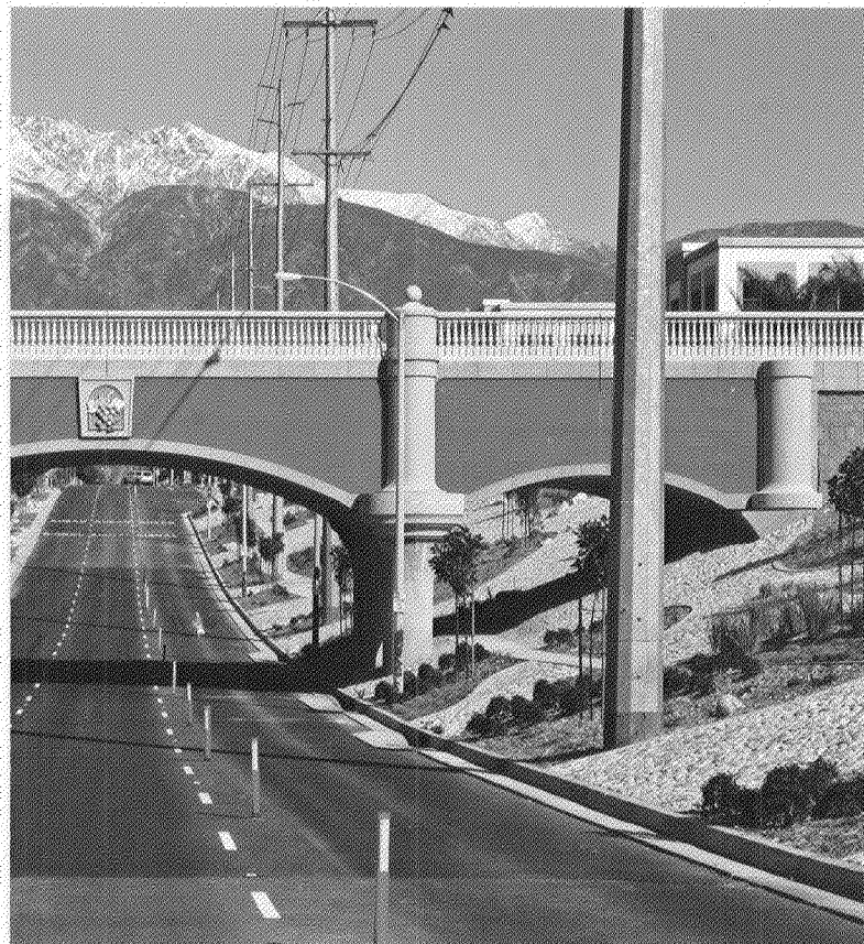
Oldcastle Precast developed prestressed concrete post-tension box girders for the City of Rancho Cucamonga outside of Los Angeles, California. The bridge includes a 33-foot and a 52-foot girder, together carrying two railroad tracks over Haven Avenue.
