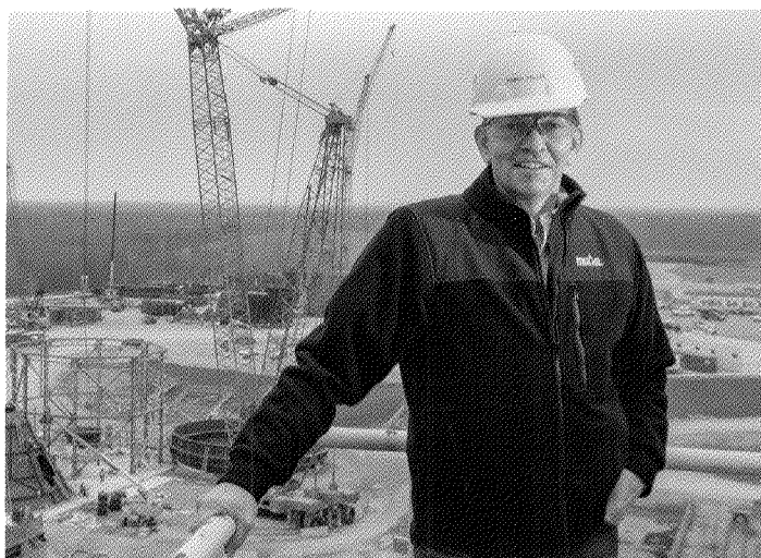
Randy Pollek, MGE's joint plant manager, oversees MGE's interests at the Columbia Energy Center in Portage, Wis., where scrubbers, baghouses and activated carbon injection systems are being installed.
