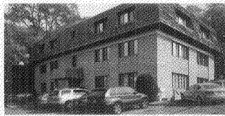
2 7 Riversville Road Greenwich, Connecticut
