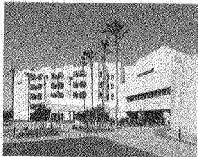
Hoag Hospital Irvine, California LEED Silver
