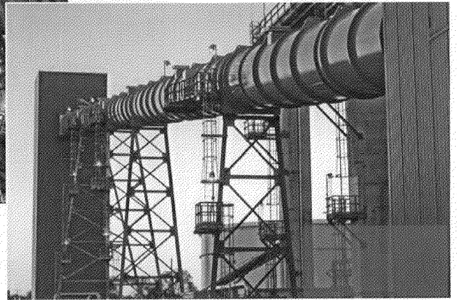
Below, coke conveyor at the Detroit refinery
