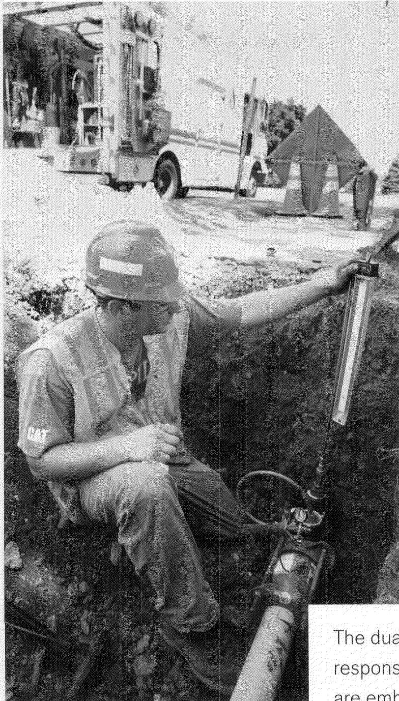
▲ Michael Argauer of the Company's Utility subsidiary inspects a low-pressure distribution line in Lackawanna, N.Y., maintaining National Fuel's commitment to operating a safe and reliable system.
