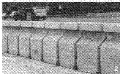
1. The Road Zipper System laterally transfers a barrier wall at speeds of up to 7 mph (11 km/h) 2. QuickChange® Moveable Barrier system
