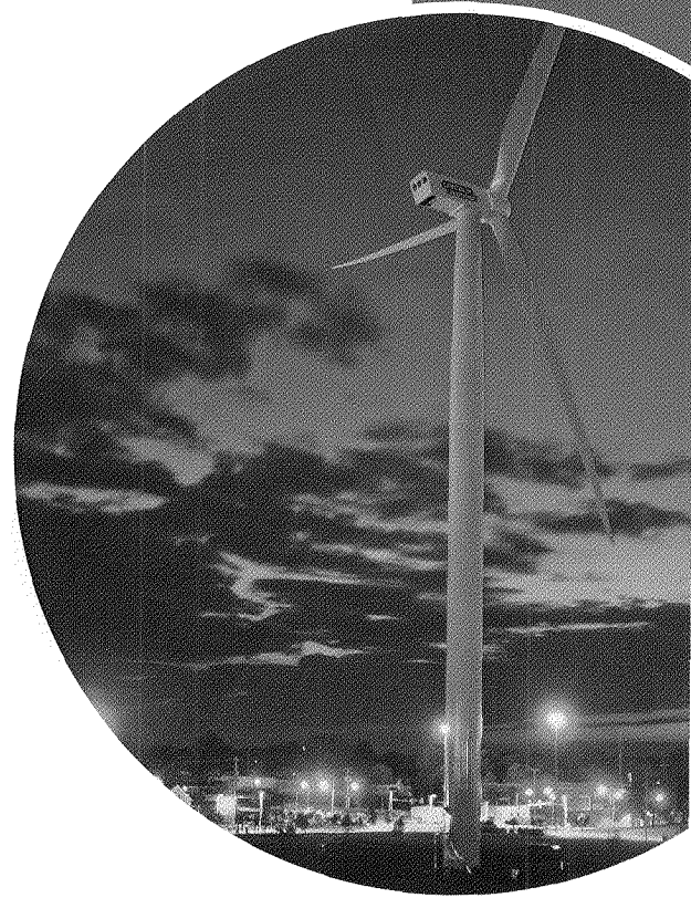
Wind tower at Lincoln's corporate headquarters in Cleveland, Ohio.
