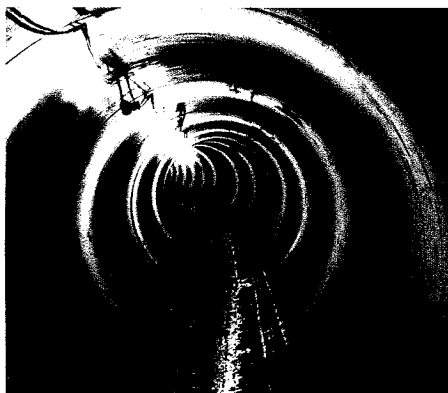
The new Albrighton sewer
