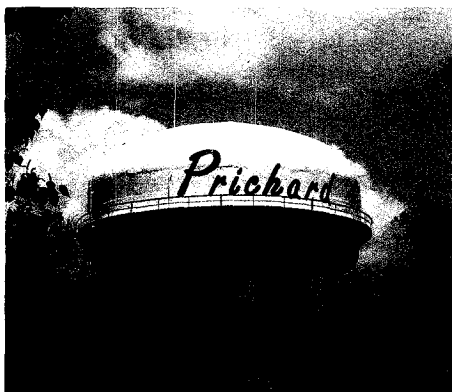
Prichard Water Tower
