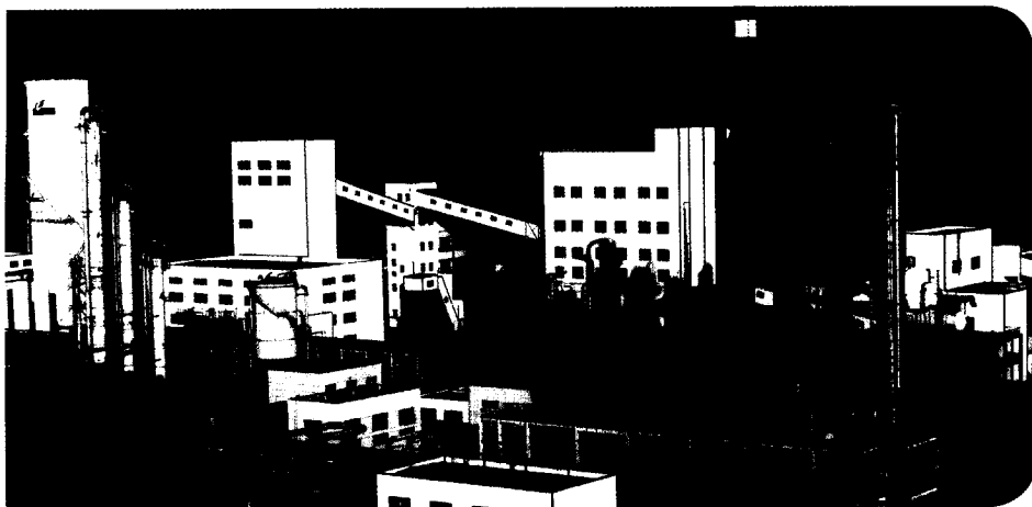
left ECO's coal-based chemical plant in Erdos, Inner Mongolia.
