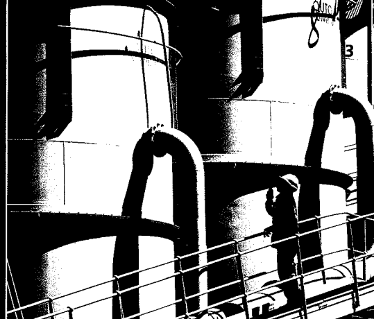
Flotation cells at the concentrator plant for Xstrata Alloys' Eland operation in South Africa
