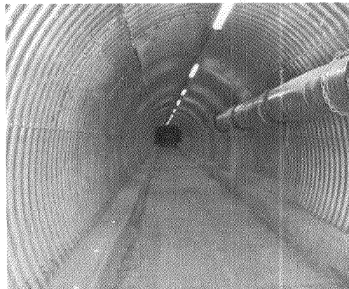
South Decline Boxcut with ARMCO-lined steel sets
