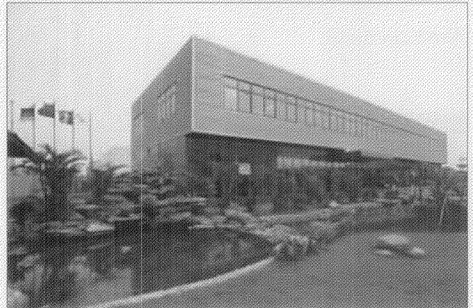
Foshan, China New Jewellery & Electroplating production and recycling facility
