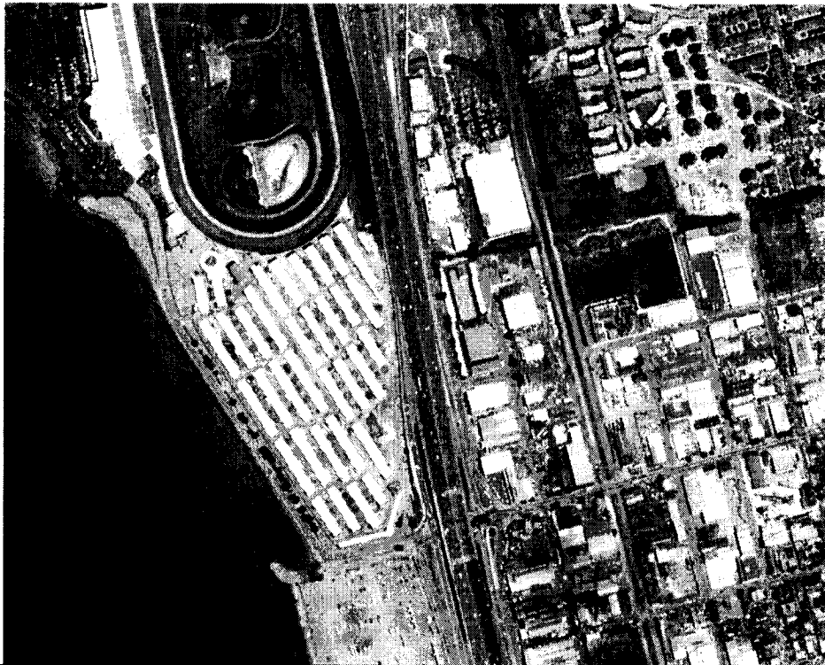
AERIAL VIEW OF THE STABLES
