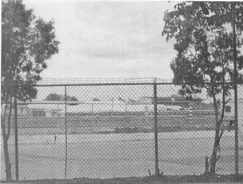
TYPICAL VIEW OF THE SUBJECT (PHOTOGRAPH TAKEN MAY 2009)
