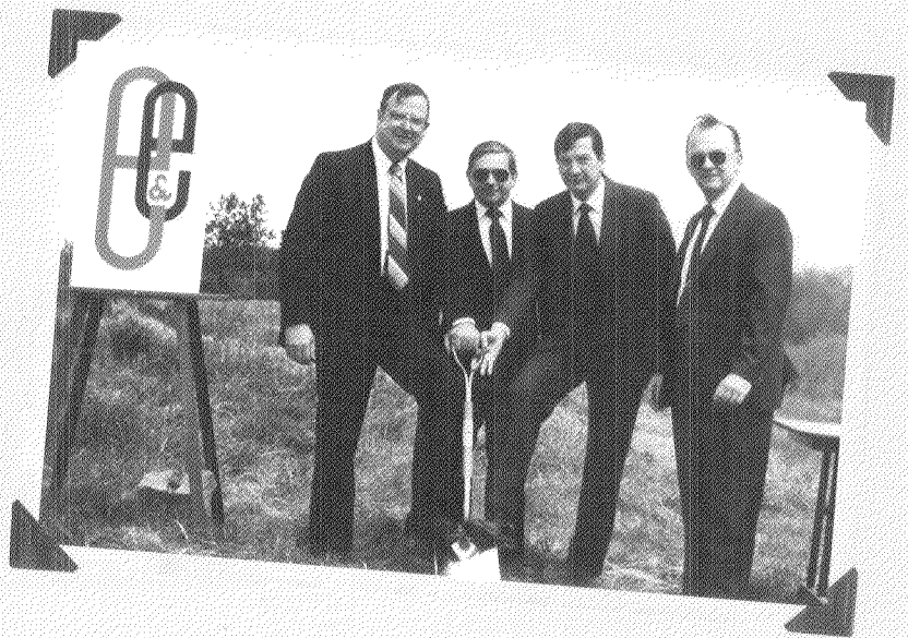
The founders (from left to right), Messrs. Neumaier, Frank, Silvestro, and Strobel, break ground for E & E's Buffalo Corporate Center in 1987.
