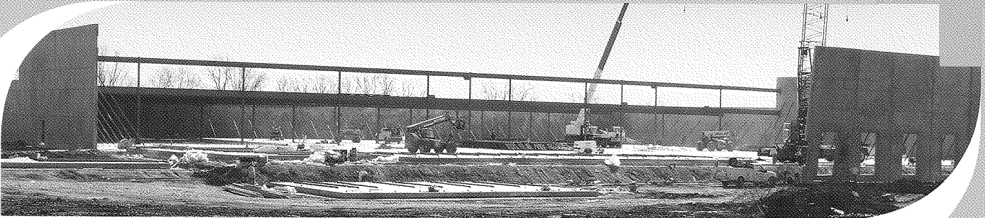
Construction of the production wing of the York facility in March 2010.
