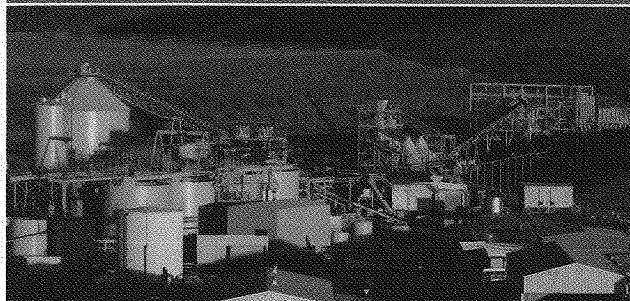
Gwalia Deeps facilities
