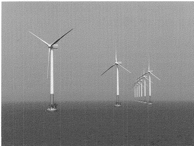
Sinovel's 3 MW Wind Turbines in Shanghai Harbor
