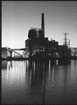
Duluth Steam District #2 is located at the Hibbard Energy Center in Duluth, Minn.
