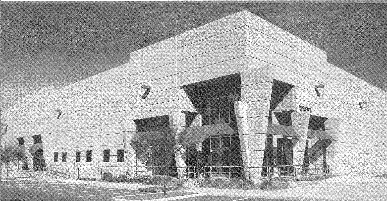
COUNTRY CLUB COMMERCE CENTER III, TUCSON, ARIZONA
