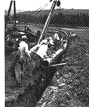
The 1937 construction of New York State Natural Gas's Line No. 8.
