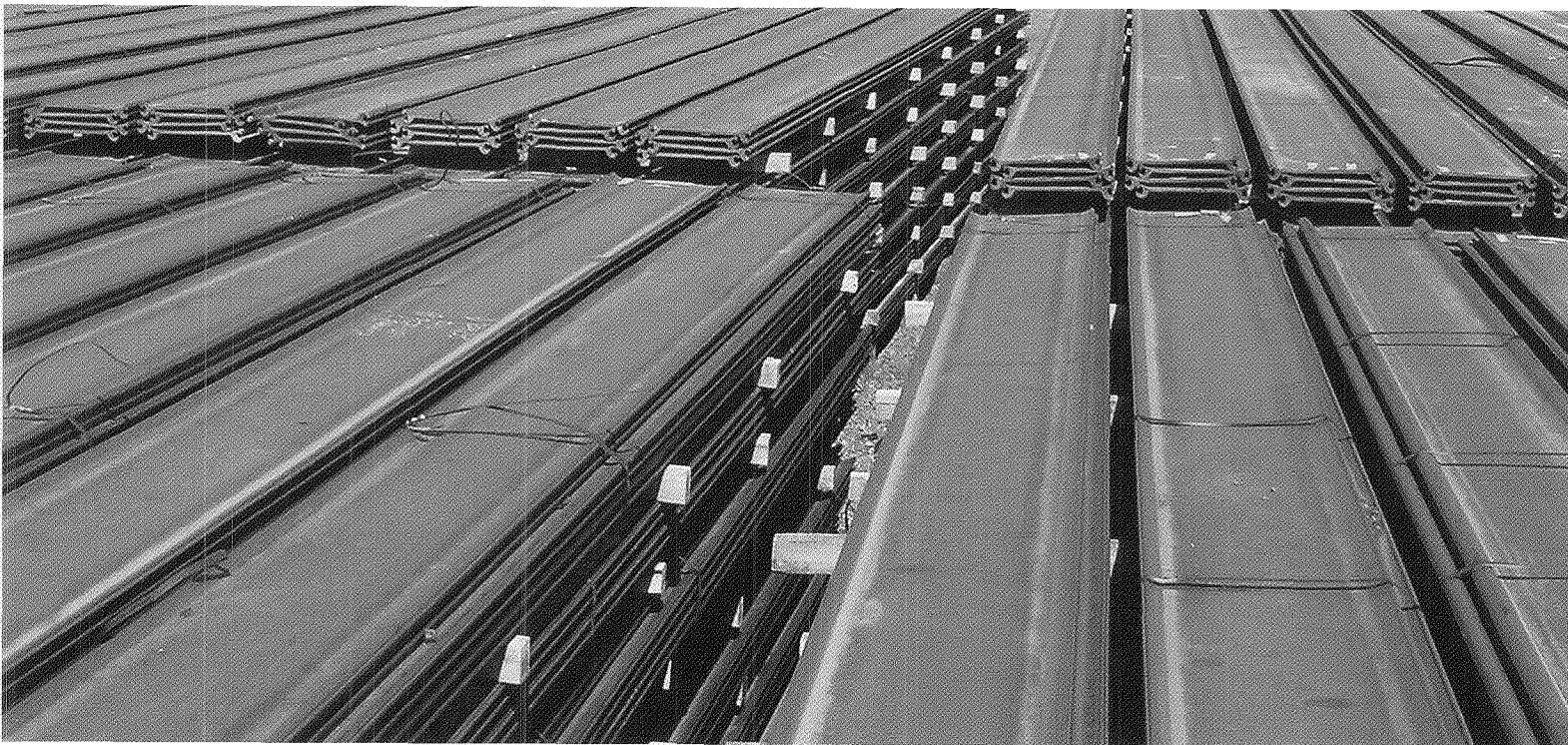
Panama Canal Expansion
