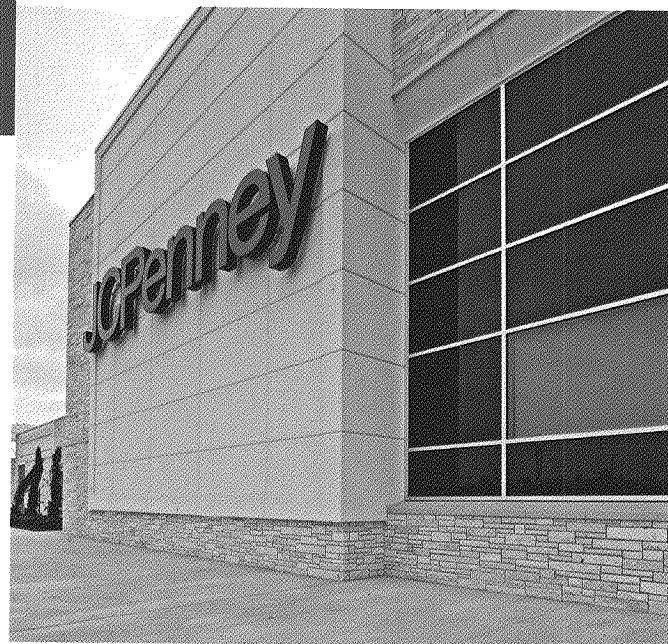
Our Fairview, Texas store was designed and constructed to achieve LEED certification from the United States Green Building Council
