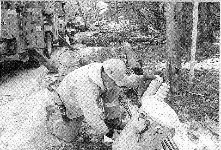
Middlebury Line Foreman Rick Canfield inspects a transformer while crews work to make repairs behind him following the December storm.
