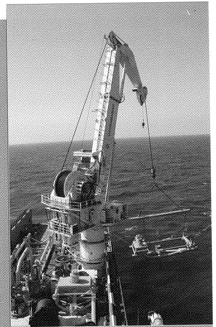
Pipeline Tie-In Foundation Installation
