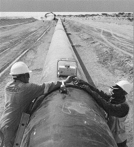
Radiographic Pipeline Weld Inspection
