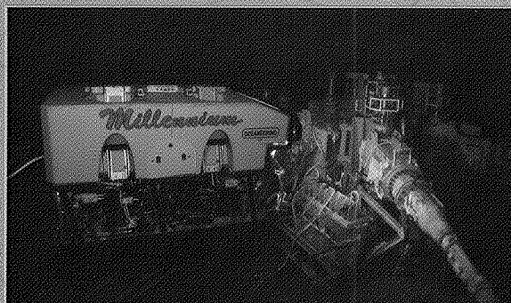
Maintenance and Repair of Electrical Hydraulic Distribution Unit
