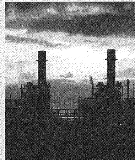
Calpine is proud to include this photo of Hidalgo Energy Center in Edinburg, TX, taken by Don Flanagan, Operator Technician I.
