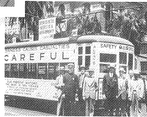
City officials with Tampa Electric's Safety Streetcar, 1928.
