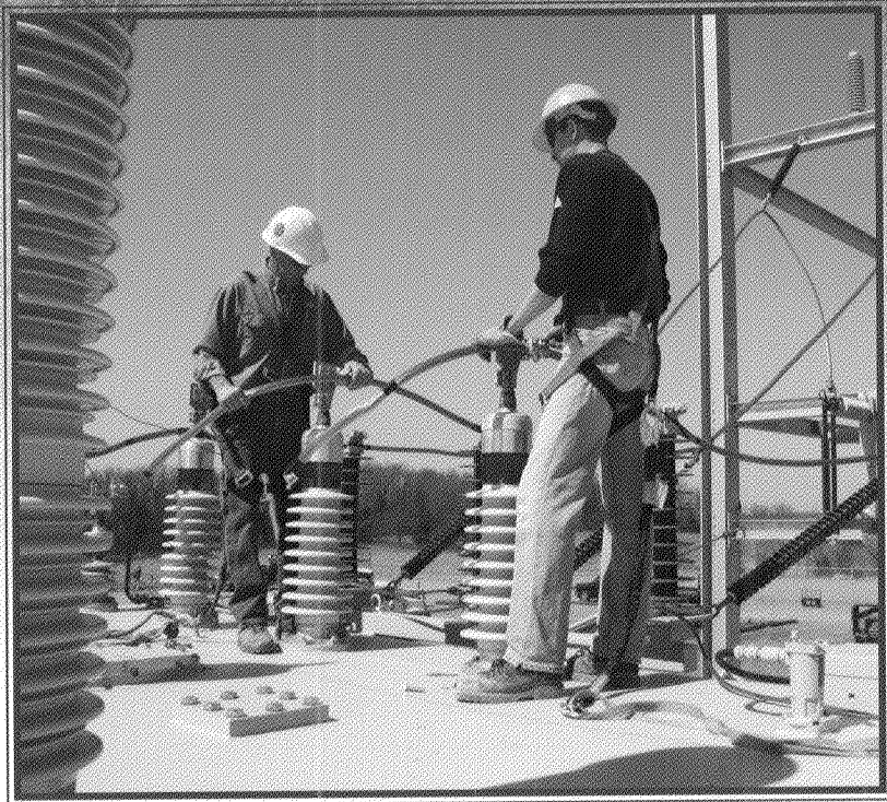
Clyde and Rusty, Substation Maintenance
