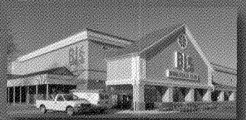
11 The Dock Stratford, Connecticut
