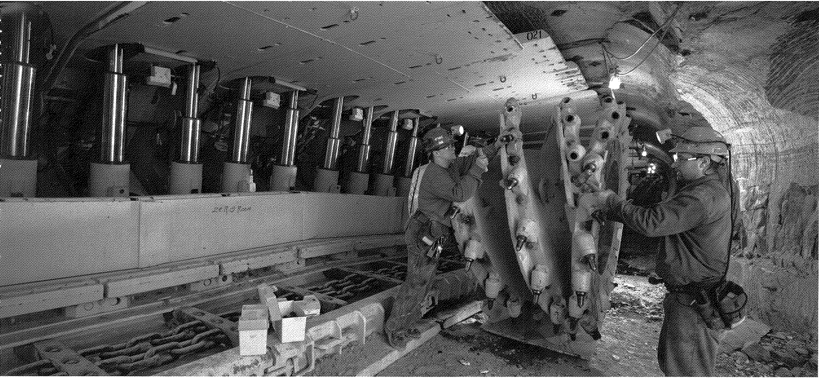
▲ FMC's Alkali Chemicals Division installed a new longwall mining system at the company's Green River, Wyo., mine in 2008. Longwall mining is nearly eight times more productive than other dry trona mining methods and provides a safer work environment. Trona is the raw material used to produce soda ash and sodium bicarbonate. Miners Heidi Hartley (left) and Monte Stoddard assemble the shearer drum of the new longwall.
