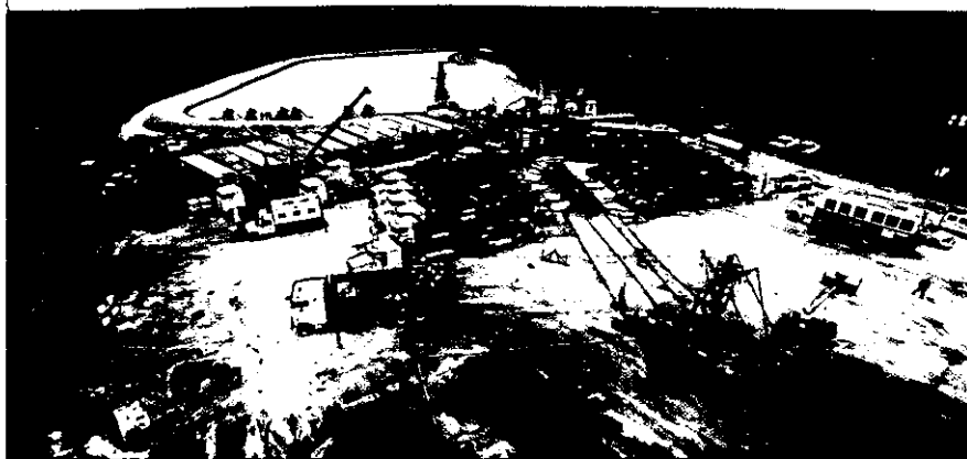
Advanced, multi-stage fracture stimulation treatments, such as this one performed on a TXCO well, hold the key to developing gas-bearing shale formations, such as the Pearsall resource play. The company placed its first Pearsall well on production in 2007 and plans to accelerate development during 2008.
