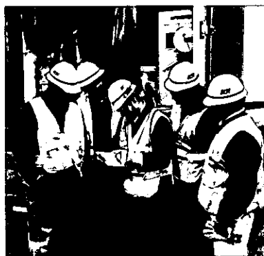
Safety is the most important part of our jobs. BGE crews, like the one shown here, begin each job by discussing safety procedures. Shown (left to right) are Dan Moser, overhead mechanic; Vernon Mitchell, cable splicer; Jason Frith, cable splicer trainee; Patrick McBurney, cable splicer; and Dave Wisniewski, senior construction inspector.
