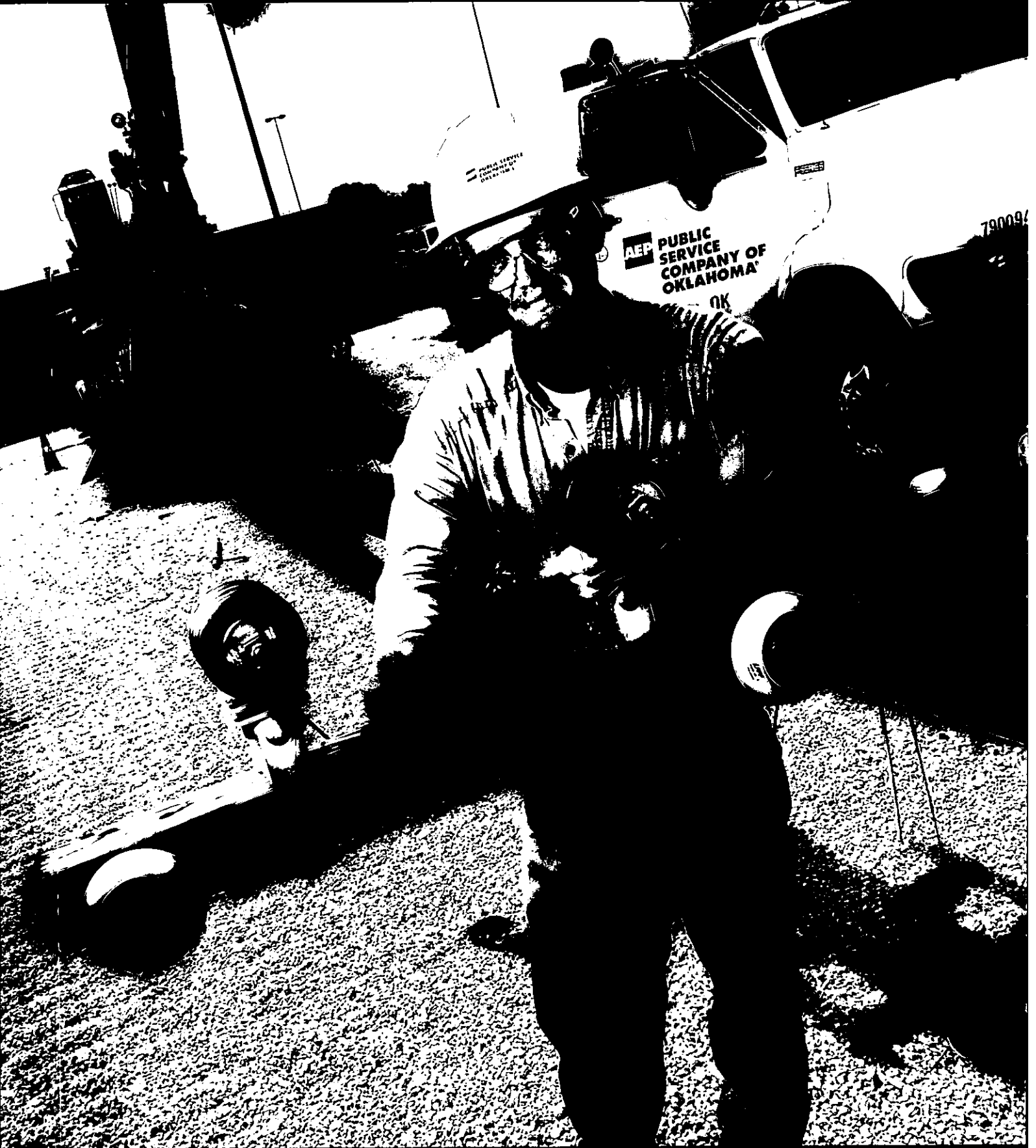
A highly skilled work force is key to the efficient, reliable operation of AEP's energy delivery facilities. Here, Ben Johannsen, journeyman line mechanic with Public Service Company of Oklahoma, works with a crew preparing to install a new distribution pole.
