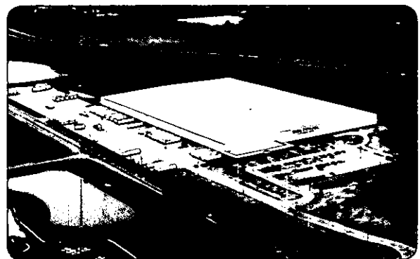
Our new Distribution Center in Evansville, Indiana.
