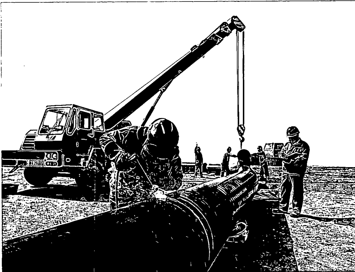
In a joint tri-partnership, Hong Kong and China Gas has participated to construct a high-pressure natural gas pipeline system in Hangzhou that will eventually supply household, commercial and industrial business customers.
