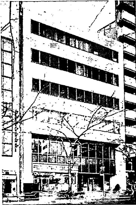
A-20 Dai-ichi Kayabacho Building
