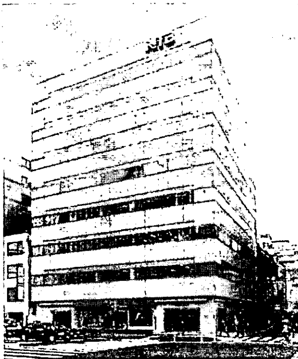
A-21 NTB · M Building
