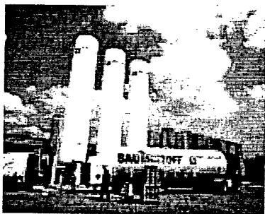
An Air Liquide unit in Germany.
