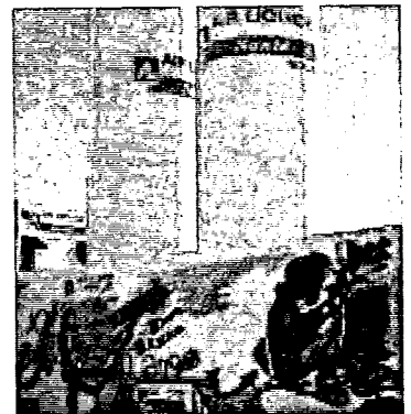
Air Liquide's site in Guadeloupe
