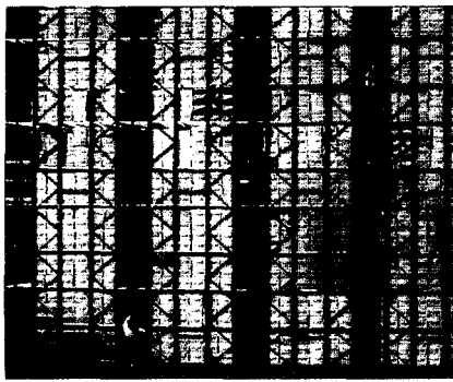
Madrid, Spain: This DMS mega-centre has the capacity to store three million cartons and is equipped with the latest fire and security measures.
