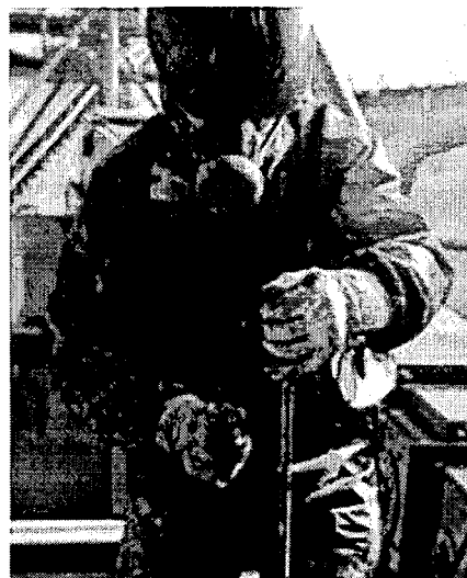
A fouled hull and propeller can increase vessel resistance in the water by 5-20%. During a docking, barnacles and other marine organisms are removed from the underwater hull and a new coat of tin-free antifouling applied.
