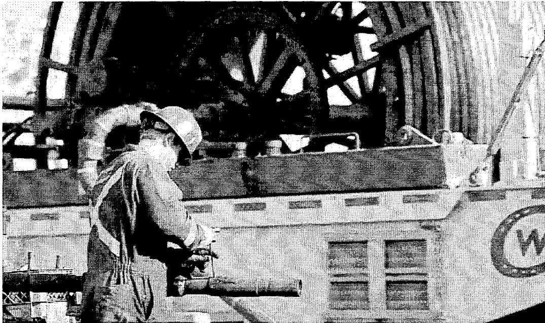
~ Highly trained field personnel conduct thorough quality control inspections of each aspect of set up and assembly, thereby ensuring the safe and successful completion of the project. Here, a Calfrac field technician assembles a specialized down hole tool for use in a fracturing through coil operation.
